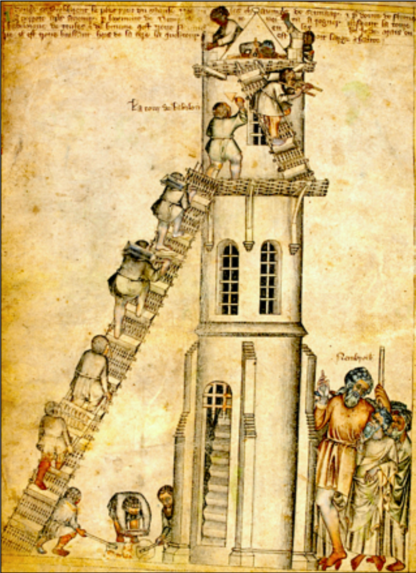
THE BRITISH LIBRARY EGERTON MM 1894, PRODUCED DURING 3RD QUARTER OF THE 14TH CENTURY, IS A CYCLE OF 149 ILLUSTRATIONS DRAWN WITH INK AND COLOR WASHES. FOLIO 5 VERSO SHOWN HERE REVEALS THE HAZARDOUS WORKING CONDITIONS OF THE TIME. THREE WORKERS BENEATH THE WOVEN WOOD LADDER ARE MIXING MORTAR FROM SLAKED LIME (CALCIUM HYDROXIDE) SAND, AND ADDITIVES OF MANY DIFFERENT KINDS DEPENDING ON REGIONAL AVAILABILITY, WHOSE COMMON PROPERTY WAS STRONGLY BONDED MOLECULAR CHAIS SUCH AS CASEIN, ANIMAL FAT, OR EGG ALBUMIN.
