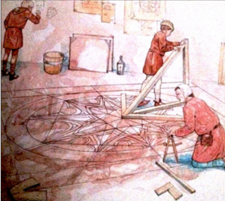
MEN TRACING DESIGN FOR STAINED GLASS ROSE WINDOW USING THE SIMPLE GEOMETRIC DESIGN TOOLS AVAILABLE AT THE TIME SUCH AS RULERS, SQUARES, CALIPERS, AND THE PYTHAGOREAN EQUATION FOR CALCULATING AN UNKNOWN LENGTH IF ONE HAS THE LENGTHS OF THE RIGHT-ANGLED SIDES.
