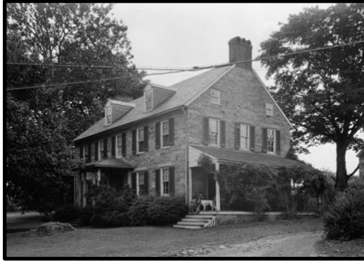
Kirk House Darlington, Maryland 13
